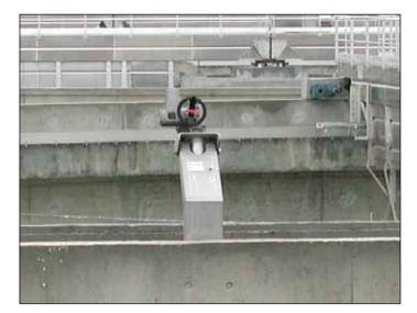
of hot-galvanised steel as standard. Side plates and the spindle protective casing are made of stainless steel.
