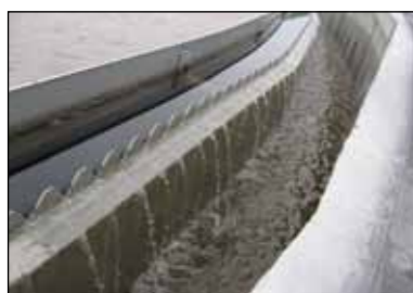
Betonrende med: KD 16.17 Flydeslamskant. KD 16.14 Hakkant.
